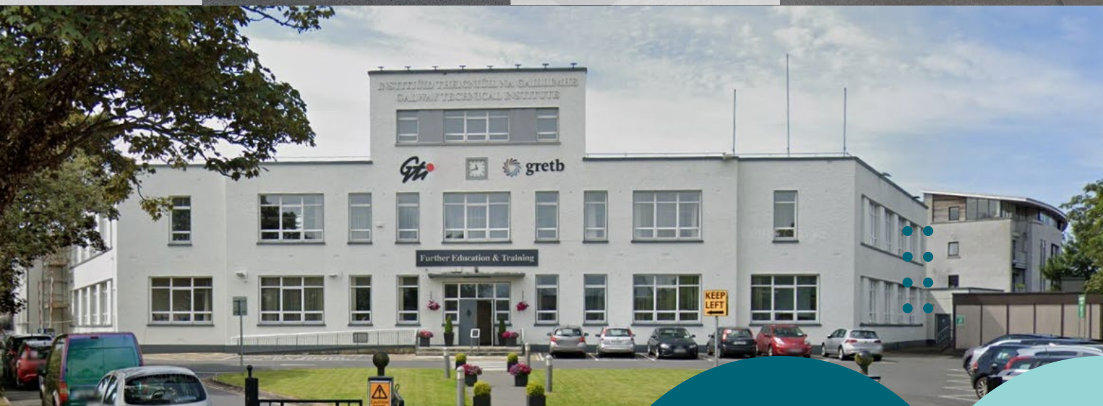
Galway Technical Institute (GTI) had an upgrade of the heating centre which included replacing old oil boilers with new condensing gas boilers. A refurbishment of the existing roof was completed. An upgrade of fire alarm and emergency lighting to comply with current standards was installed. Universal access toilets and external ramps were completed.
