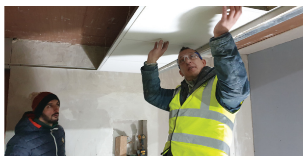
Tipperary ETB Dry Lining Class
