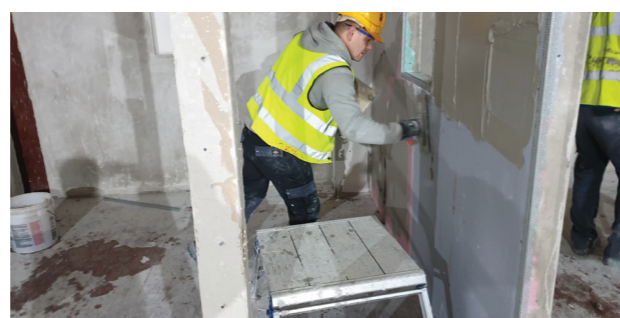
Tipperary ETB Dry Lining Class
