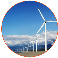
Wind Turbine Maintenance
